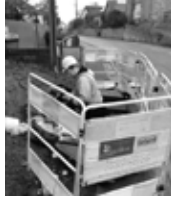
Stage 2 - Jan 17th, connection testing?
